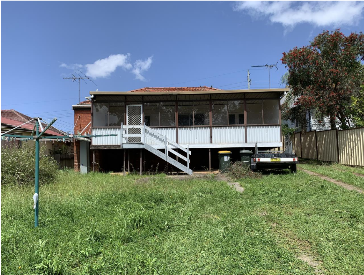
Figure 12. The rear of the site building had an enclosed steel paneled and glass verandah with a wooden staircase that led to the rear garden.
