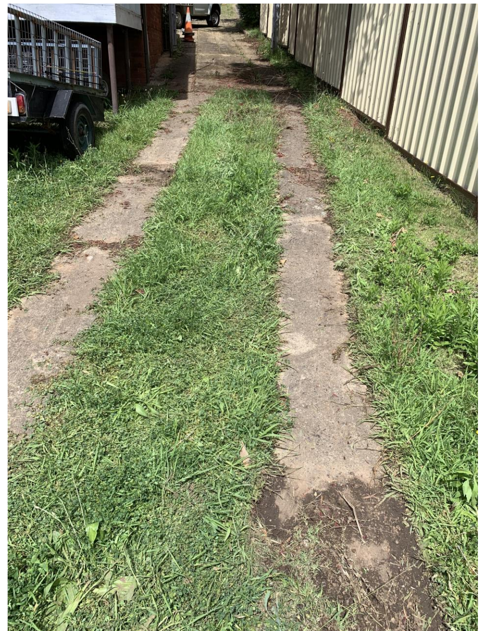
Figure 17. The driveway transitioned from entirely concrete to concrete with grass through the center within the rear of the site. The concrete was persistently degraded along the length of indicating the driveway segments are the same age.
