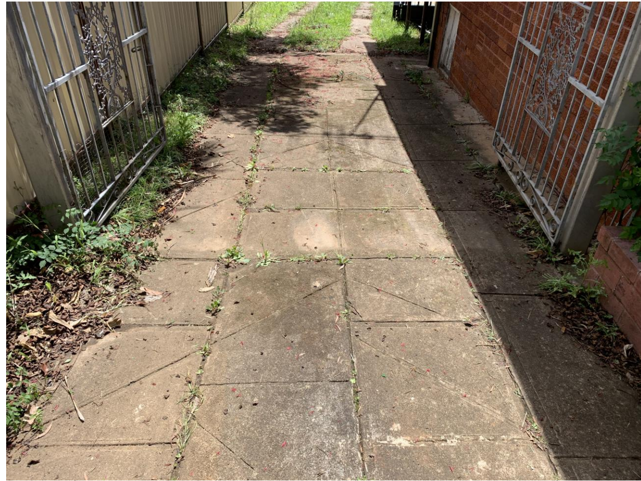
Figure 11. A degraded concrete driveway extended along the western perimeter from the road, through double metal gates and into the rear of the site.
