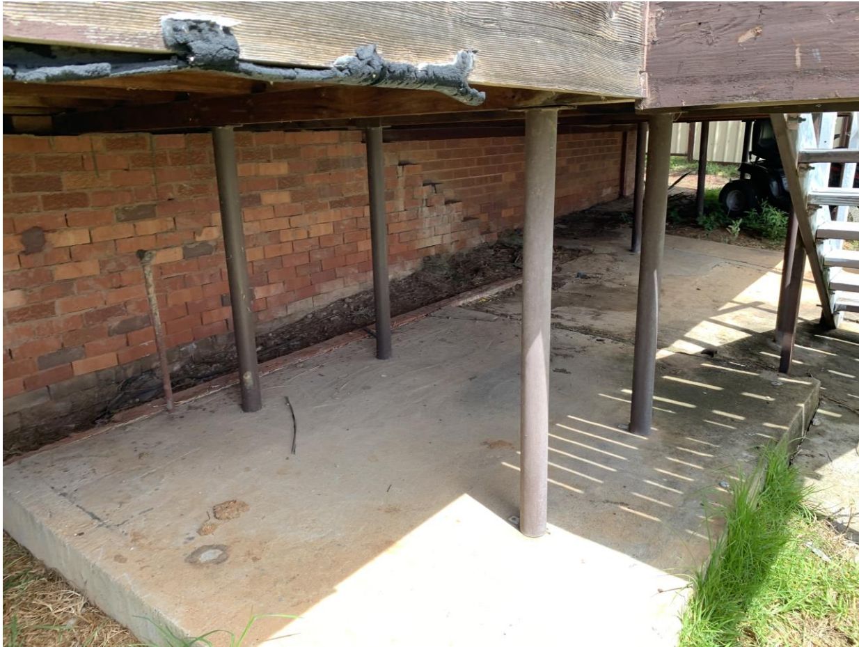
Figure 14. Beneath the verandah. The verandah was built on stilts and concrete slab.
